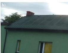
**Fig. 3.** Typical forms of external condensation of water vapor on envelopes: a) on the glass facade; no condensation in the upper part of the room and near poorly insulated structural frames, b) on the roof slope; no condensation in places of poorly insulated rafters (*own photos*)
