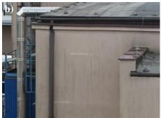
**Fig. 4.** Permanently soiled facades with acrylic plaster. Unsoiled surfaces in the area of: a) mounting pins, b) gaps between the panes (*own photos*)
