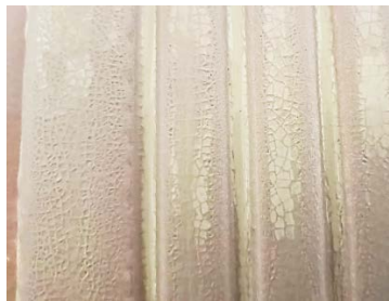
Fig. 7. Cracks on the surface of the experimental brick samples with engobe No. 2 after firing at 950°C ( own research )
