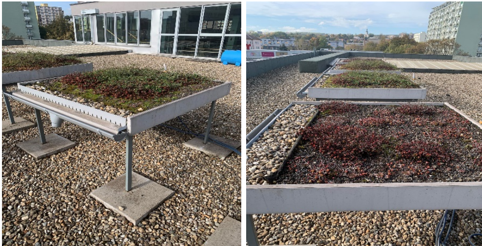
Fig. 4. Experimental areas of green roofs, Technical University of Košice ( own photo )
