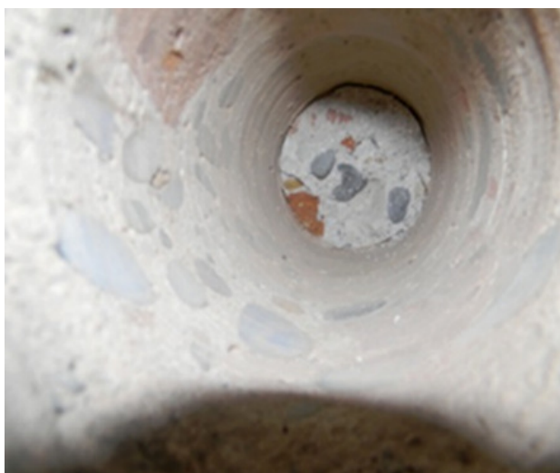
Fig. 3. Lightweight concrete mix obtained in forced mix concrete ( own research )
